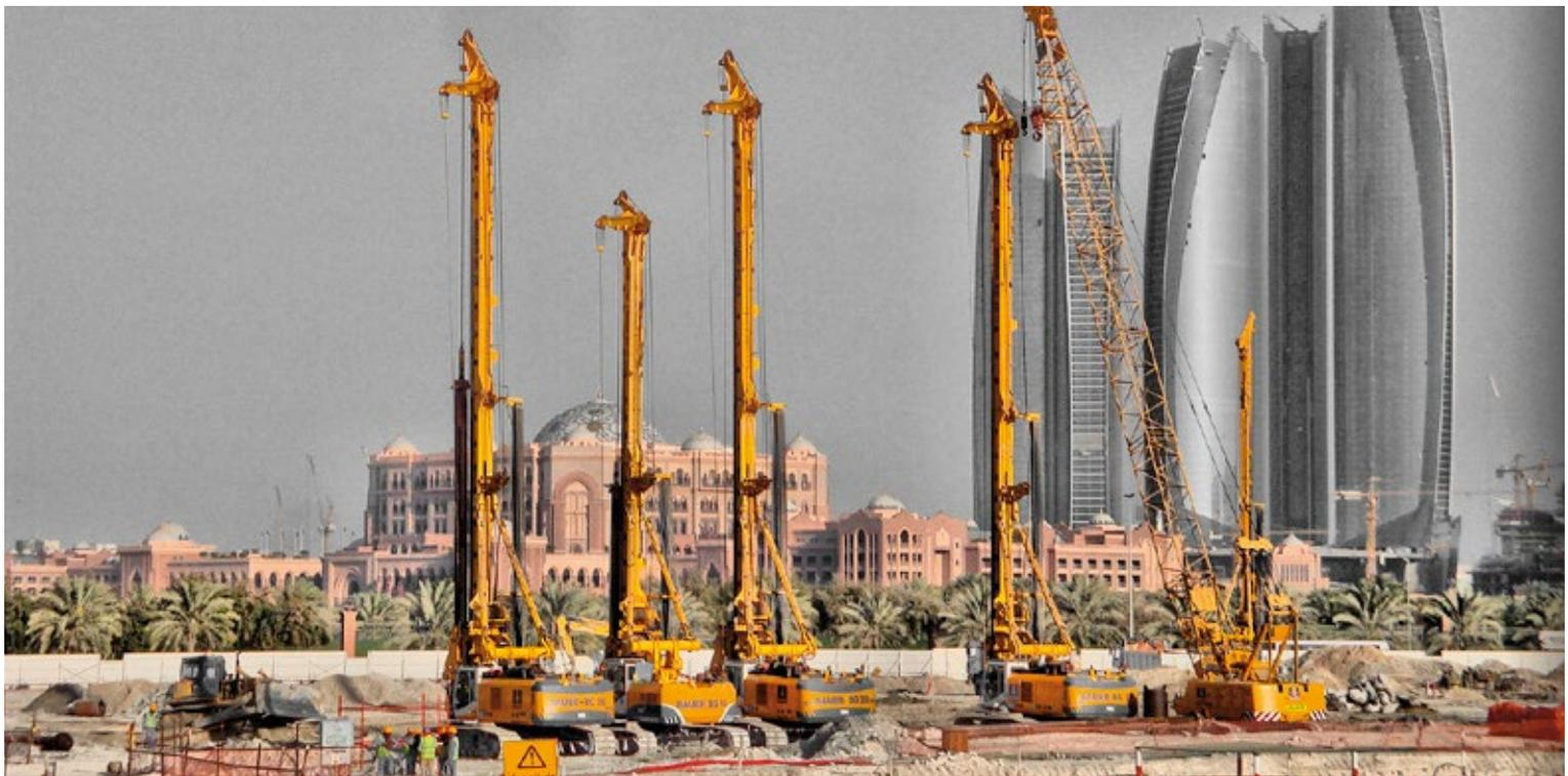
Presidential Palace in Abu Dhabi: one of BAUER's prestige projects. Most of the heavy-duty rotary drilling rigs are custom-made for each construction project.
